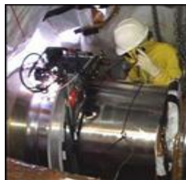
Primary Piping Replacement
